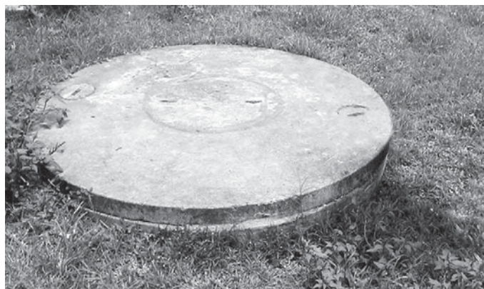
The lid of a concrete septic tank.
