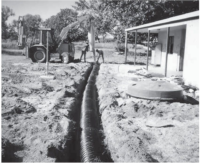
A new absorption trench being installed.
