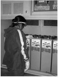
Battery banks pose a serious electrocution threat, as well as the risk of sulphuric acid burns and hydrogen gas explosion. Battery maintenance should be carried out by qualified technicians familiar with requirements for safety equipment and procedures. For a battery larger than 115V, a qualified electrician is required for all work.
