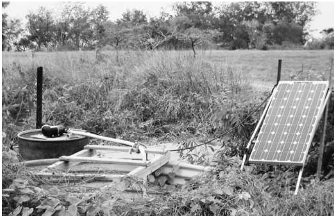
Solar-coupled diaphragm pump in shallow well, Far North Queensland.
