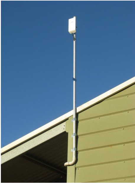
Figure 4 – Antenna mounting variations
