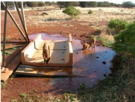
Photos 6 and 7: The area under the storage tank was often flooded and participants built an outflow pipe and concrete trough.
