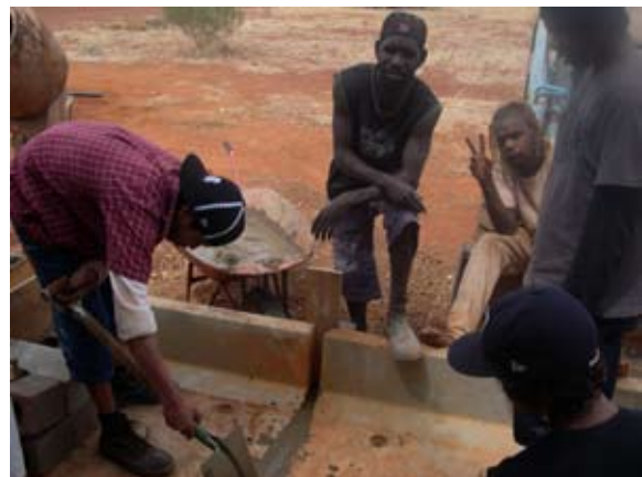
Photos 6 and 7: The area under the storage tank was often flooded and participants built an outflow pipe and concrete trough.
