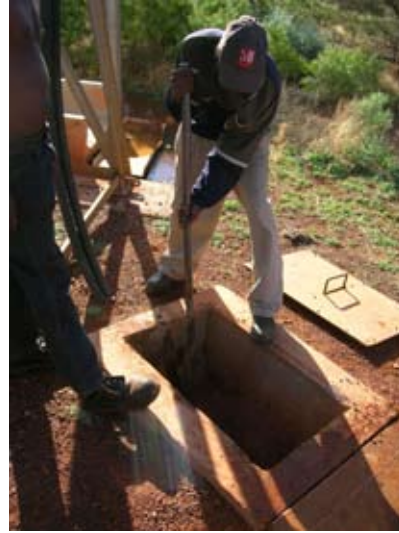
Photos 8 and 9: Participants concreted around the base of the storage tank and created a channel to direct any overflow away from the settlement. A flow valve was fitted to the main tank.
