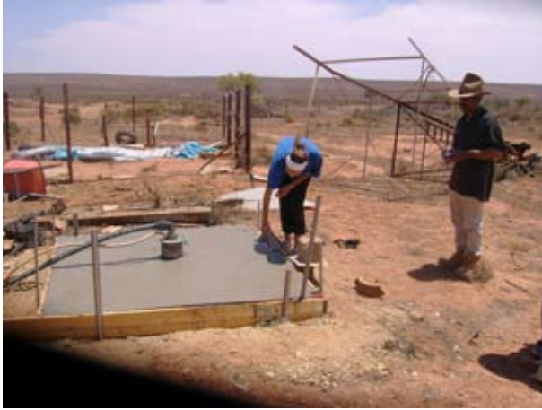
Photos 2 and 3: A concrete apron and fence were built to protect the borehead. A water meter was also installed at the bore. Leaking pipes were fixed.
