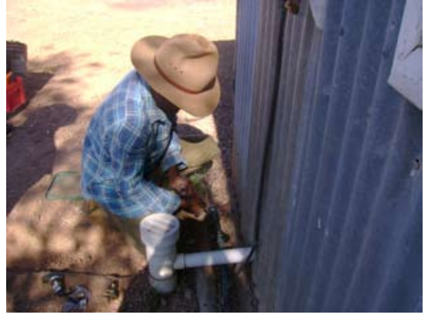
Photos 2 and 3: A concrete apron and fence were built to protect the borehead. A water meter was also installed at the bore. Leaking pipes were fixed.
