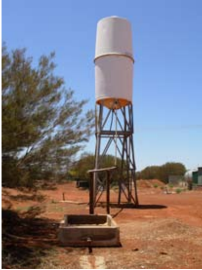
Photos 8 and 9: Participants concreted around the base of the storage tank and created a channel to direct any overflow away from the settlement. A flow valve was fitted to the main tank.
