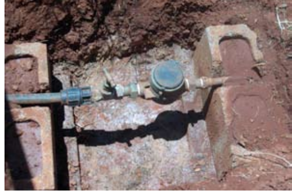
Photo 3: Water meters were fitted at the bore and at each house.
