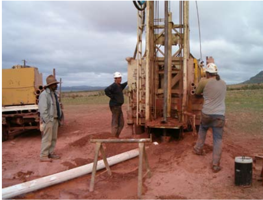
Photo 1: Drilling the bore at Yappala, June 2004
