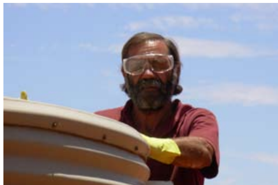
Photo 2: Reg disinfects a rainwater tank.
