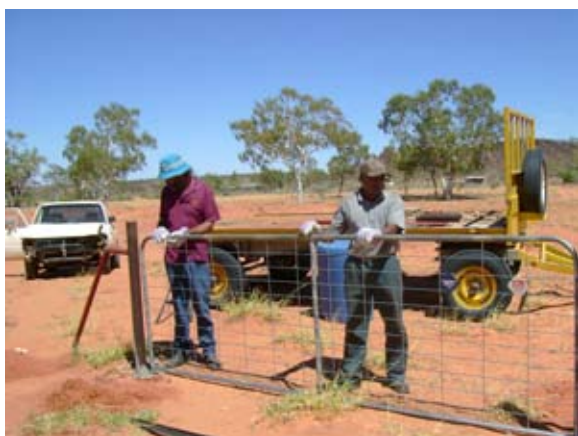
Photos 3 and 4: A fence was built around the bore and pump to protect it from cars and wandering stock.
