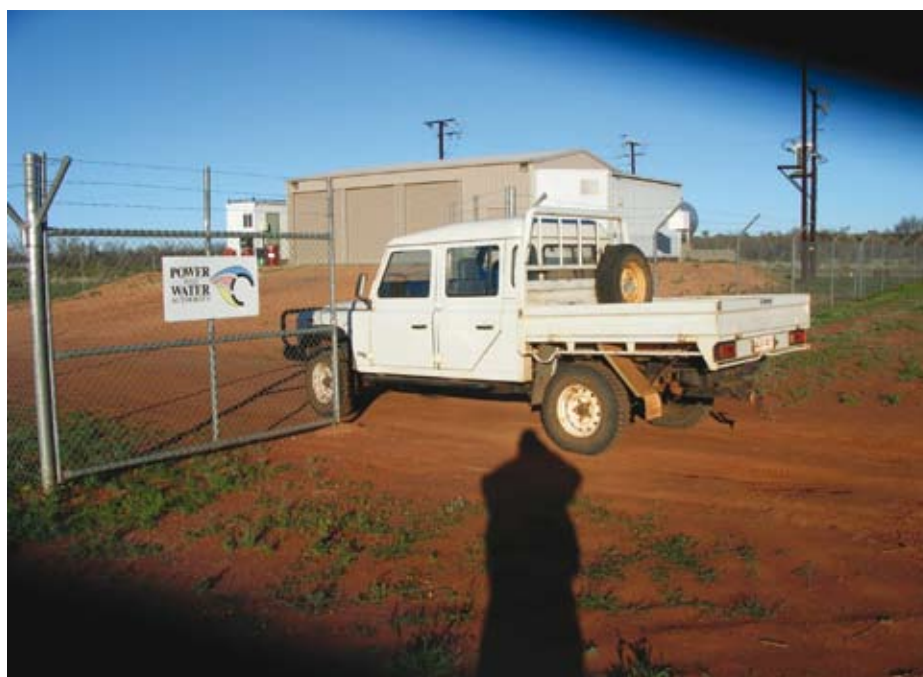
Figure 26: Engawala power station
