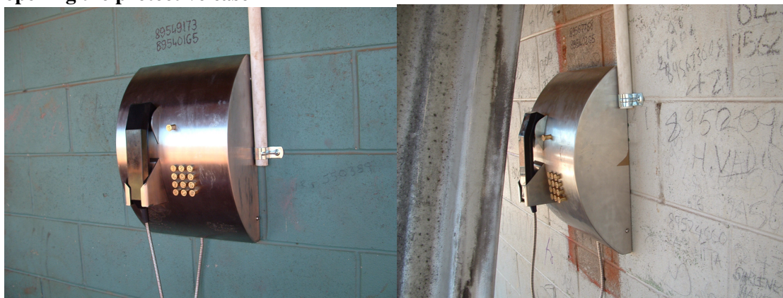
Picture 3 & 4: Phones lines entering Community Access Telephone which impinges on opening the protective case
