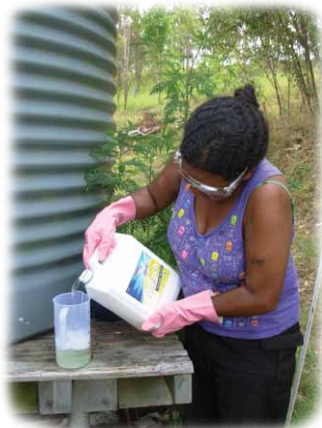
Bleach treatment of rainwater tanks.
