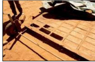
Brick making for construction
